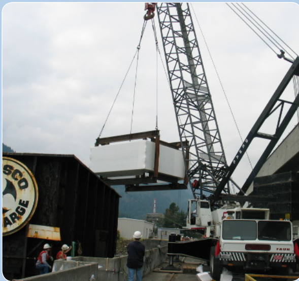
FIGURE 3. The finished prototype production antenna during its delivery to Bonneville Dam.
