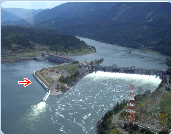
FIGURE 1. Aerial photo of Bonneville Dam taken by the U.S. Army Corps of Engineers. The arrow points to the straight section of the exit flume for the new corner-collector bypass system where the PIT-tag antennas will be installed.
